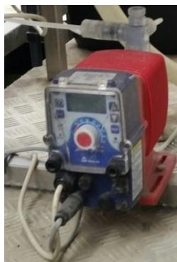
Figure 5-1. Dosage pump (the pump, tubes, etc. have to be resistant to the corrosive character of the chemicals)
