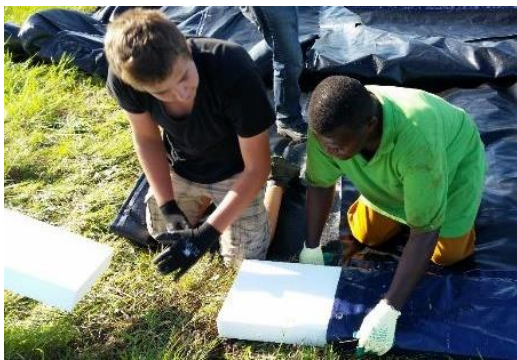
Figure 2-31. Installing the floats (Source: PSKW)
