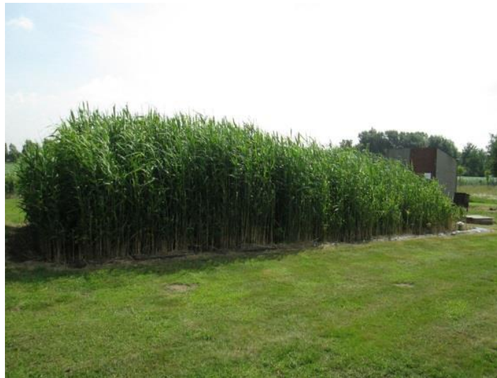
Figure 12-12. Horizontal flow wetland at PCS (Belgium)
