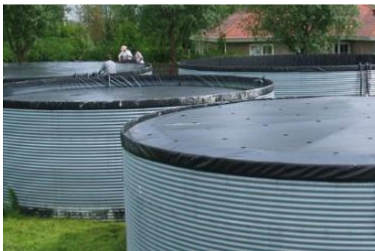
Figure 2-26. Fixed cover stretched over a water silo
