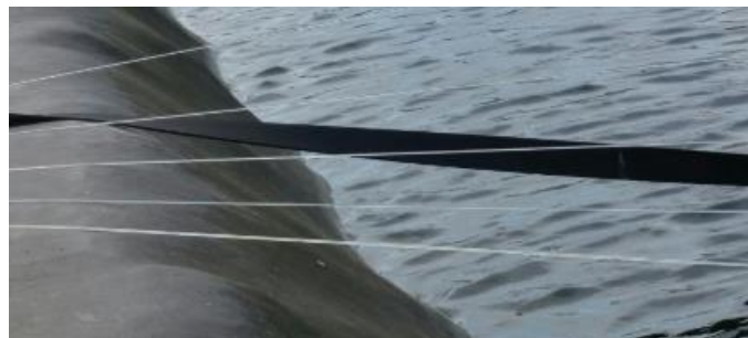
Figure 2-28. Atlas cords can be a tool to prevent water birds from landing on the floating covers (Source: Els Berckmoes)
