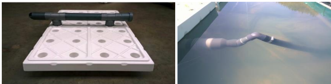
Figure 9-19. Specific float for rainwater collection (left). Connection to the rainwater storage (right) ( www.teeltdegronduit.nl )
