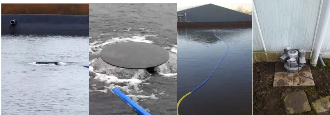
Figure 6-19. Airlift installation
