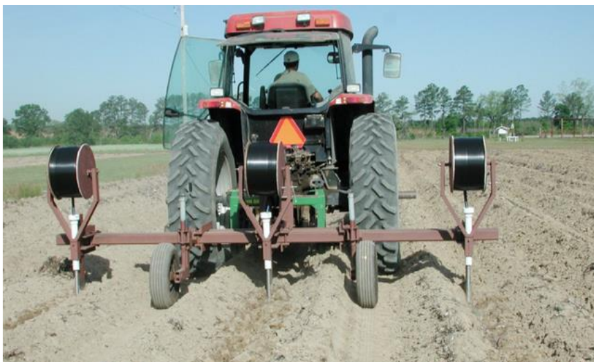
Figure 7-14. Equipment used to install the drip lines (Payero et al., 2006)
