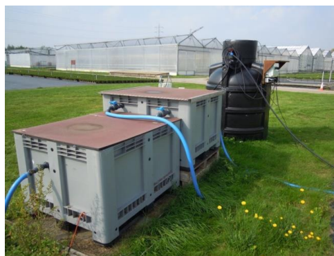
Figure 12-8. MBBR at PCS (Belgium)
