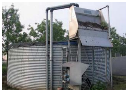
Figure 6-16. Picture of a slow sand filter (Belgium) with a sieve bend to get rid of coarse organic material before disinfecting it with the slow sand filter
