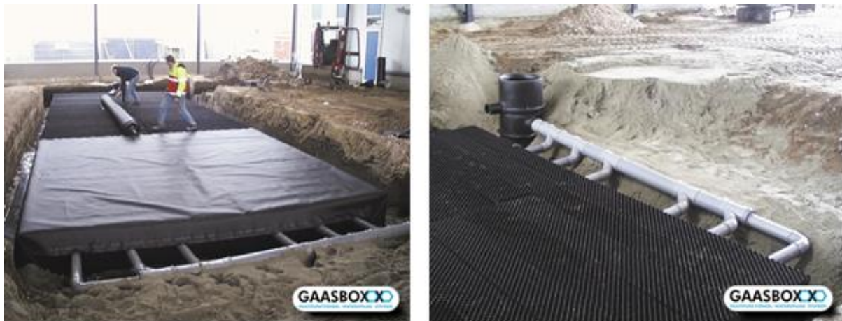
Figure 2-14. Installation of Gaasboxx ( https://jesproducts.nl/gaasboxx-systeem.htm )
