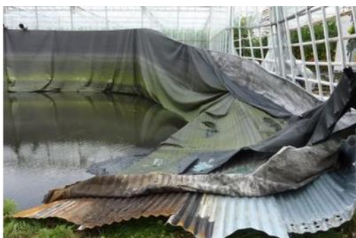
Figure 2-9. A silo has cracked due to corrosion of the lower plates ( http://www.hyente.com/nieuws.html )
