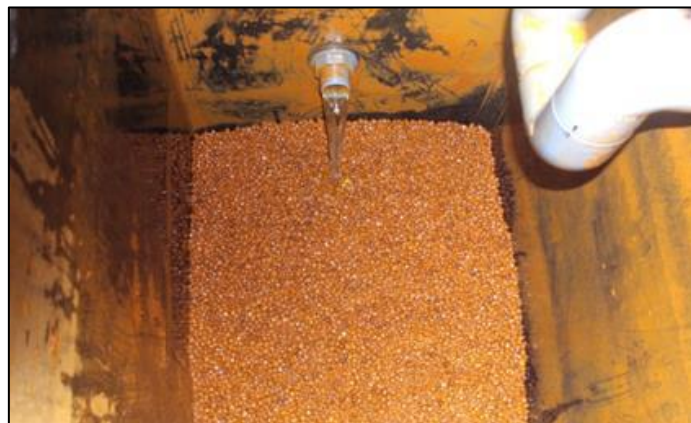
Figure 12-2. Phosphate filter based on granular iron with a sand core
